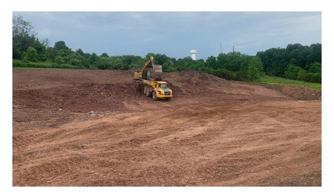
Excavation, the project's first major operation to accommodate the Turnpike widening, is ongoing on both sides in cleared areas at the northern end of the work zone, between mileposts A41.5 and A43.5, where the construction barrier is installed. Excavation and grading of sediment basins 15 and 16 on the southbound side also is currently underway (*see above*).
